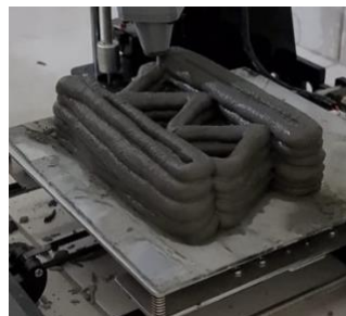
Figure 62. Hollow wall printed structure
