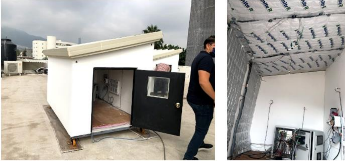
Fig 4. 5. Actual site photos of interior and exterior view of the units
