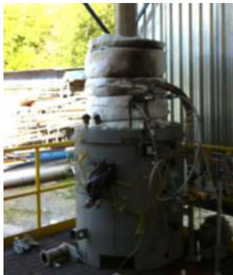
Figure 5. Solar thermal energy storage prototype and experimental setup
