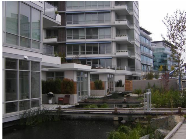
Fig. 2.16. Progress of the project by October 2008.
