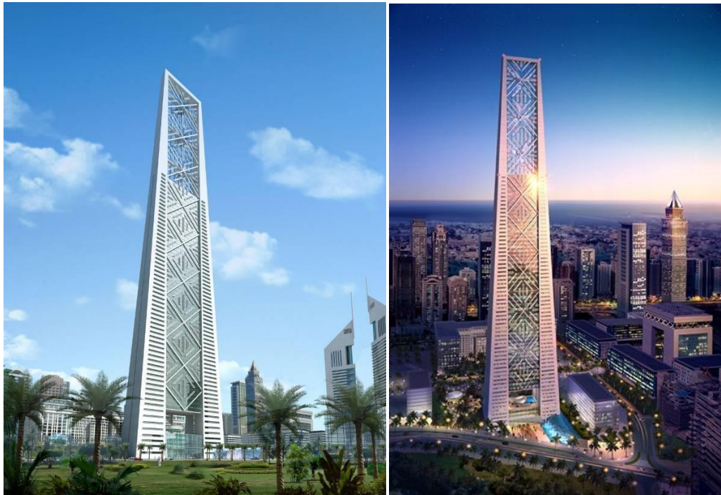
Fig. 2.7. The Lighthouse, in Dubai International Financial Center.
