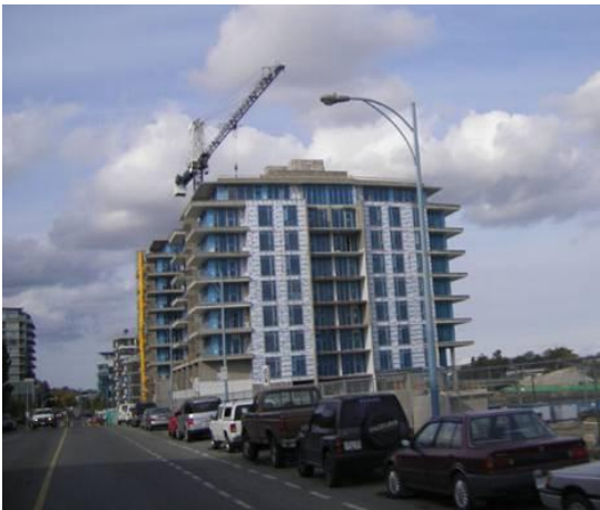
Fig. 2.15. Construction of the first phase, July 2008.
