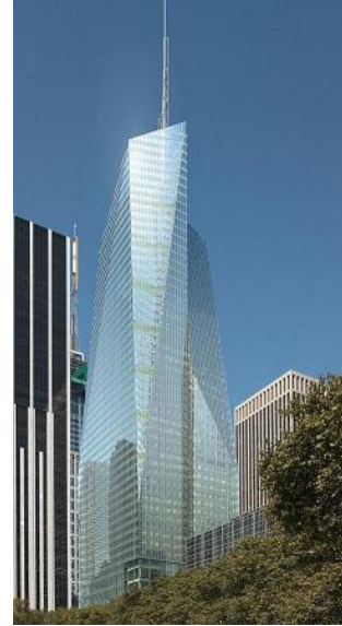
Fig. 2.11. The BoA Tower seeks to improve productivity and reduce energy consumption.
