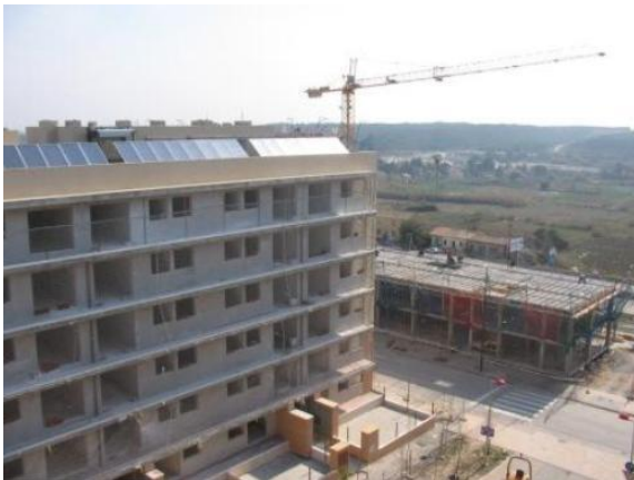
Fig. 2.21. Installation of solar panels on the rooftops.
