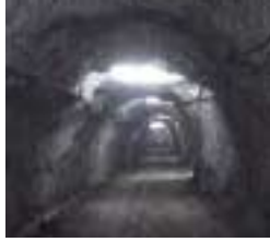
(a) Túnel Principal
