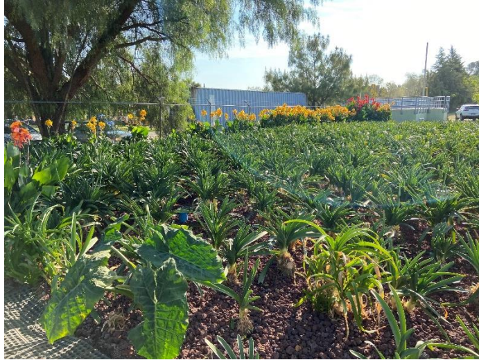
Figure 1. Horizontal flow constructed wetland (HFCW) planted with Agapanthus africanus .
